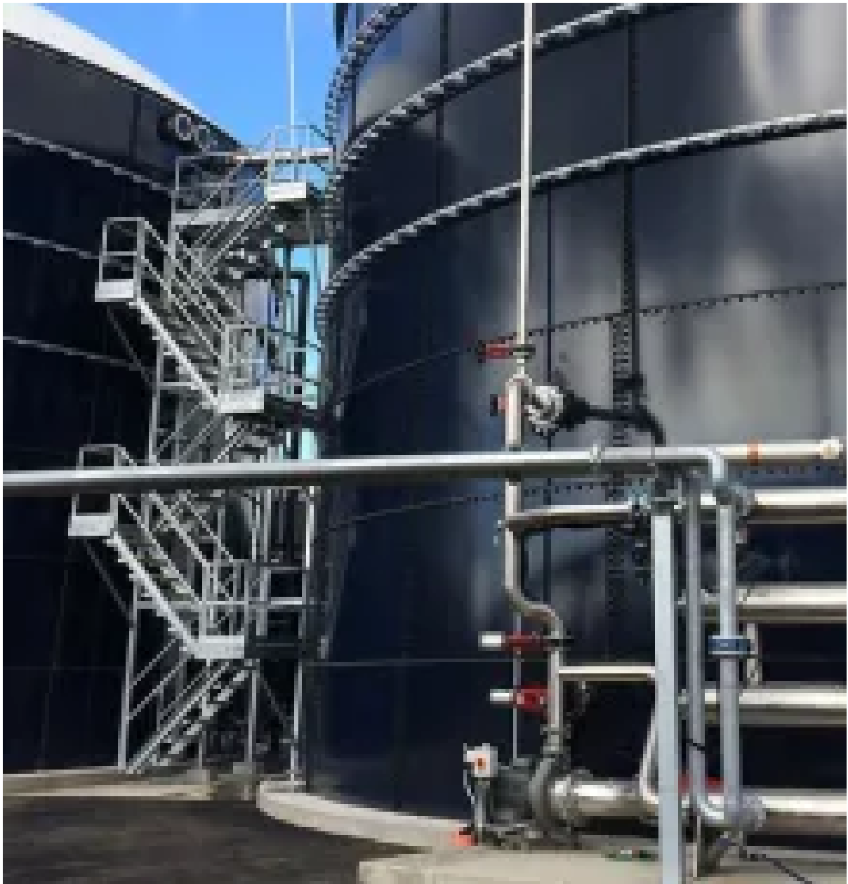
Delorean's Jandakot Bioenergy Plant in Perth. AFR
